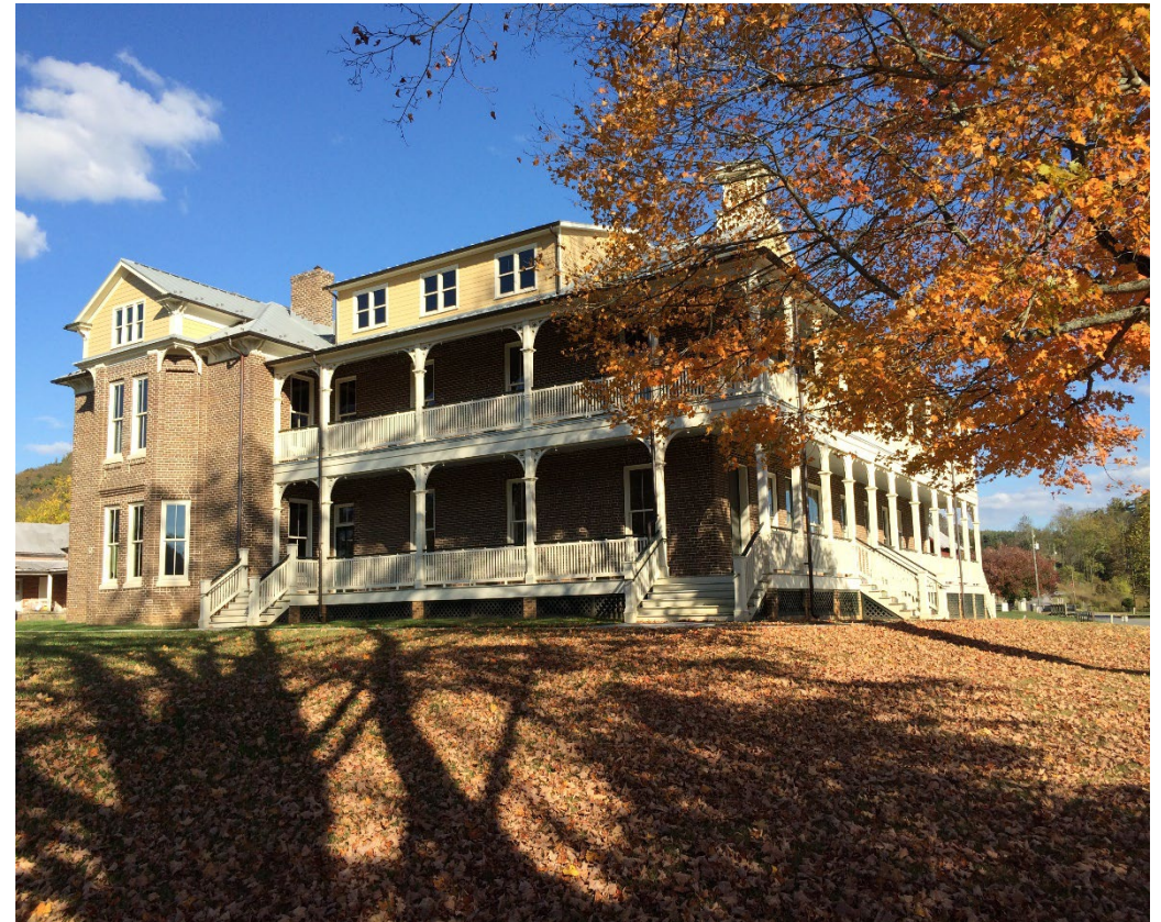
Renovation complete in 2023
